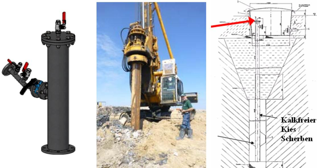
Figure 2 – Landfill gas wells (head) / drilling / complete gas well
