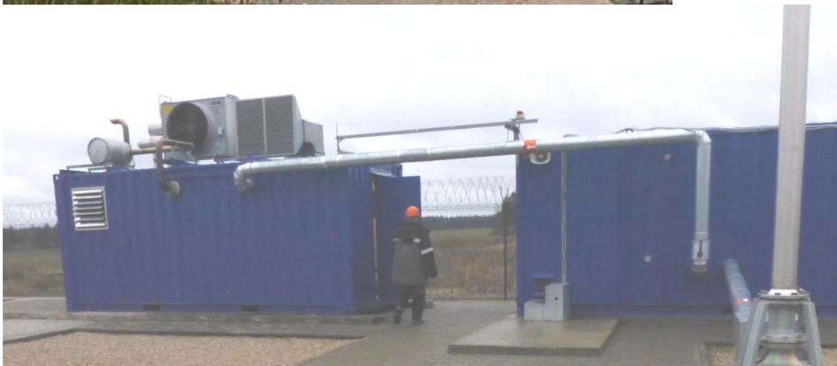
Figure 8 Containerised booster system and gensets (CHP units) Clarke Energy Ltd. in Wales (top) and Vireo in Belarus (below)
